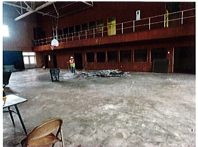
12 - DEMOLITION WORK in PROGRESS.
